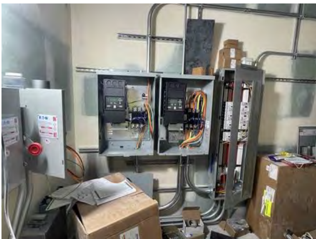
Electrical work - Penthouse panel boxes
