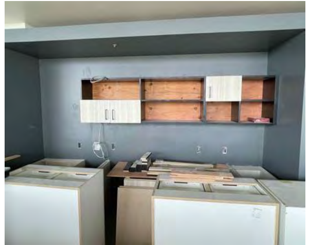
Start of PLAM cabinet install
