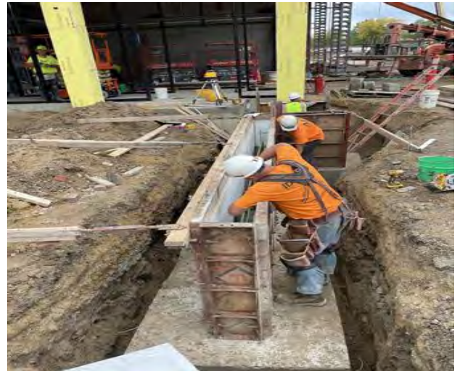
Retaining wall forming on SE corner
