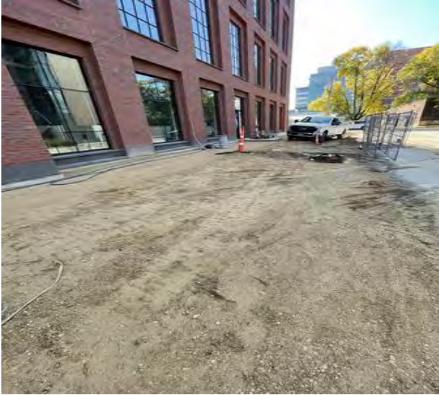
North side fill compaction / sidewalk prep
