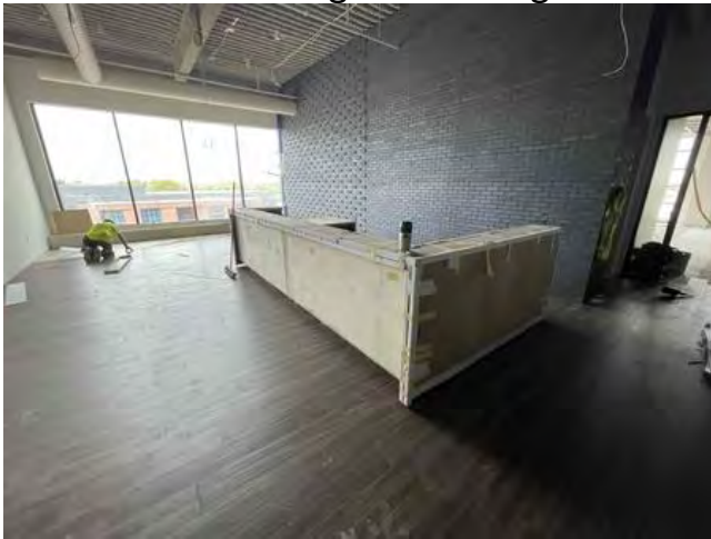
L5 flooring install & casework progress
