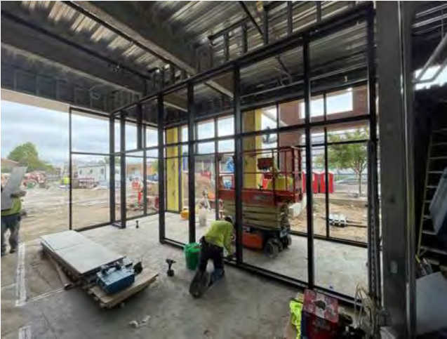
Storefront glass framing on L1
