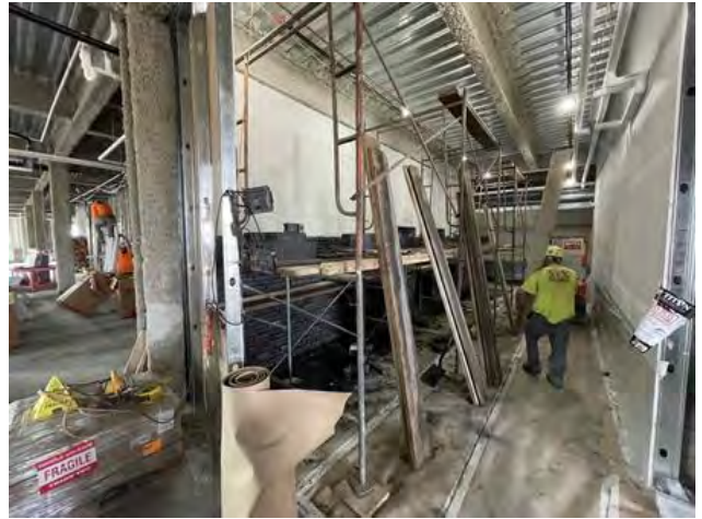
Masonry progress on L1
