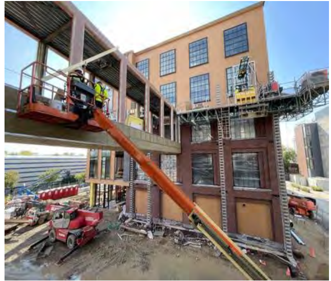
East elevation – masonry & skybridge progress
