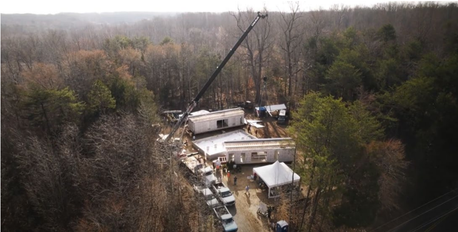
Photo courtesy of Powhatan Habitat for Humanity.
