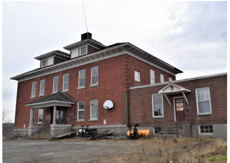
Historic Ward 5 School in Barre. Photo courtesy of Downstreet & Evernorth.
