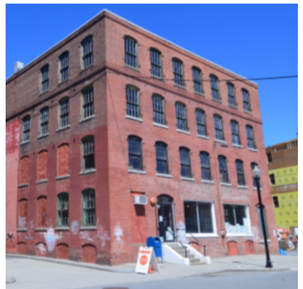
DeWitt Building in Brattleboro
