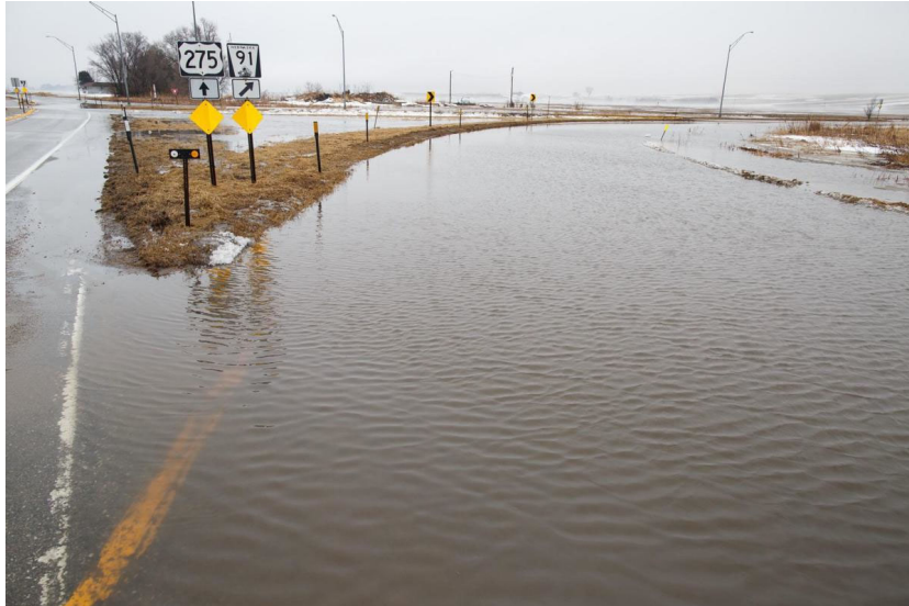
Highway 275 & Highway 91 North of Scribner, Nebraska
