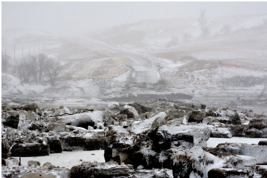
Spencer Dam Break - Holt County, Nebraska
