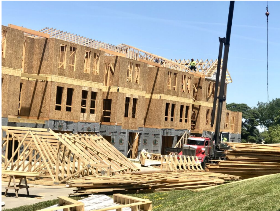
An Omaha housing construction site (Cindy Gonzalez/Nebraska Examiner)
