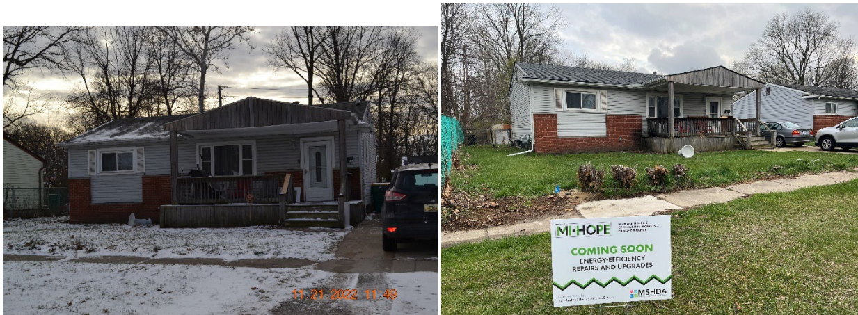
2) Before (left) and After (right): Roof and Gutter Replacement
