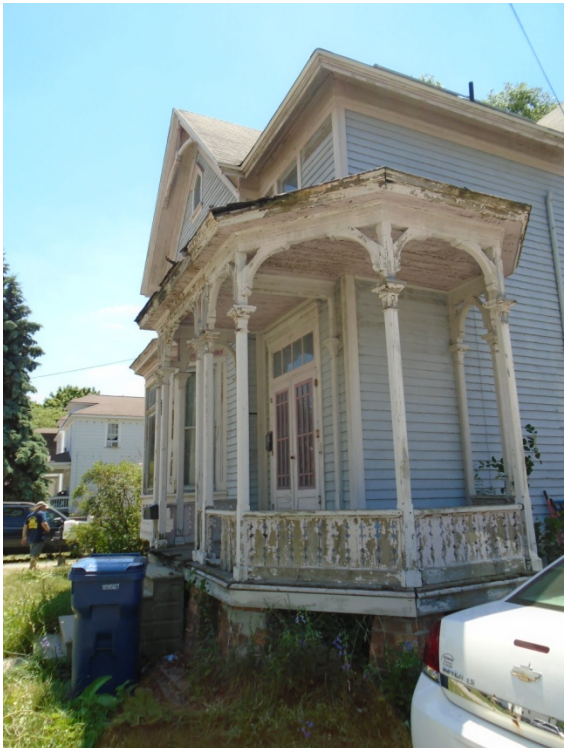
HDF-2017-5836-NEP, 521 N. Grant St., Porch Repairs BEFORE
