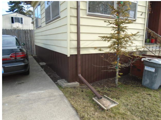
HDF-2017-5836-NEP, 510 N. Grant St., Porch Repairs AFTER
