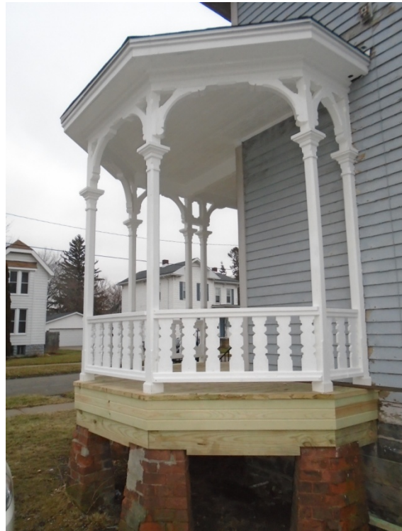
HDF-2017-5836-NEP, 521 N. Grant St., Porch Repairs AFTER
