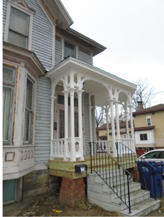
HDF-2017-5836-NEP, 521 N. Grant St., Porch Repairs AFTER
