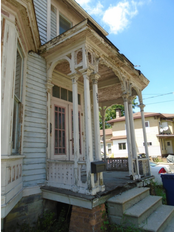
HDF-2017-5836-NEP, 521 N. Grant St., Porch Repairs BEFORE
