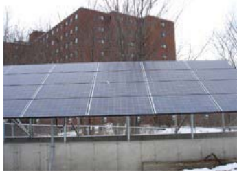
Fairweather Apartments, Salem, Massachusetts
