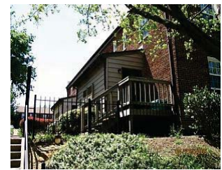
Garfield Hill Apartments, Washington, D.C.
