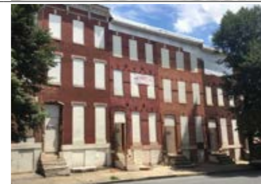
DRUID HILL AVE STABILIZATION
