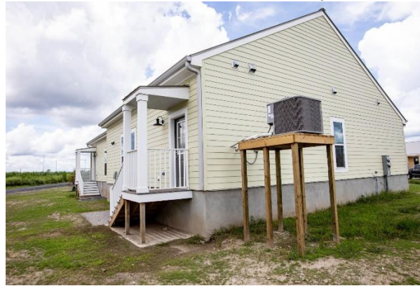
Structure with elevated HVAC systems
