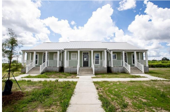
Completed front elevation
