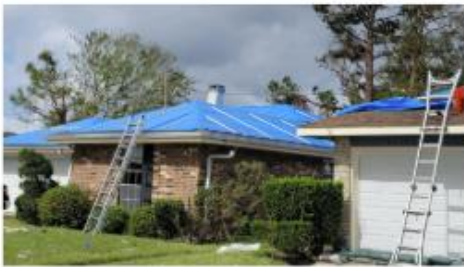
Blue Roof Installations . Courtesy of St. John the Baptist Parish
