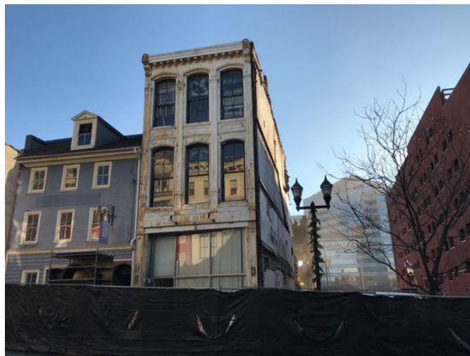
Two of the historic buildings on Market Street in downtown Wilmington that are set to be demolished for a new apartment building built by the Buccini/Pollin Group (Photo: Jeanne Kuang/ The News Journal )
