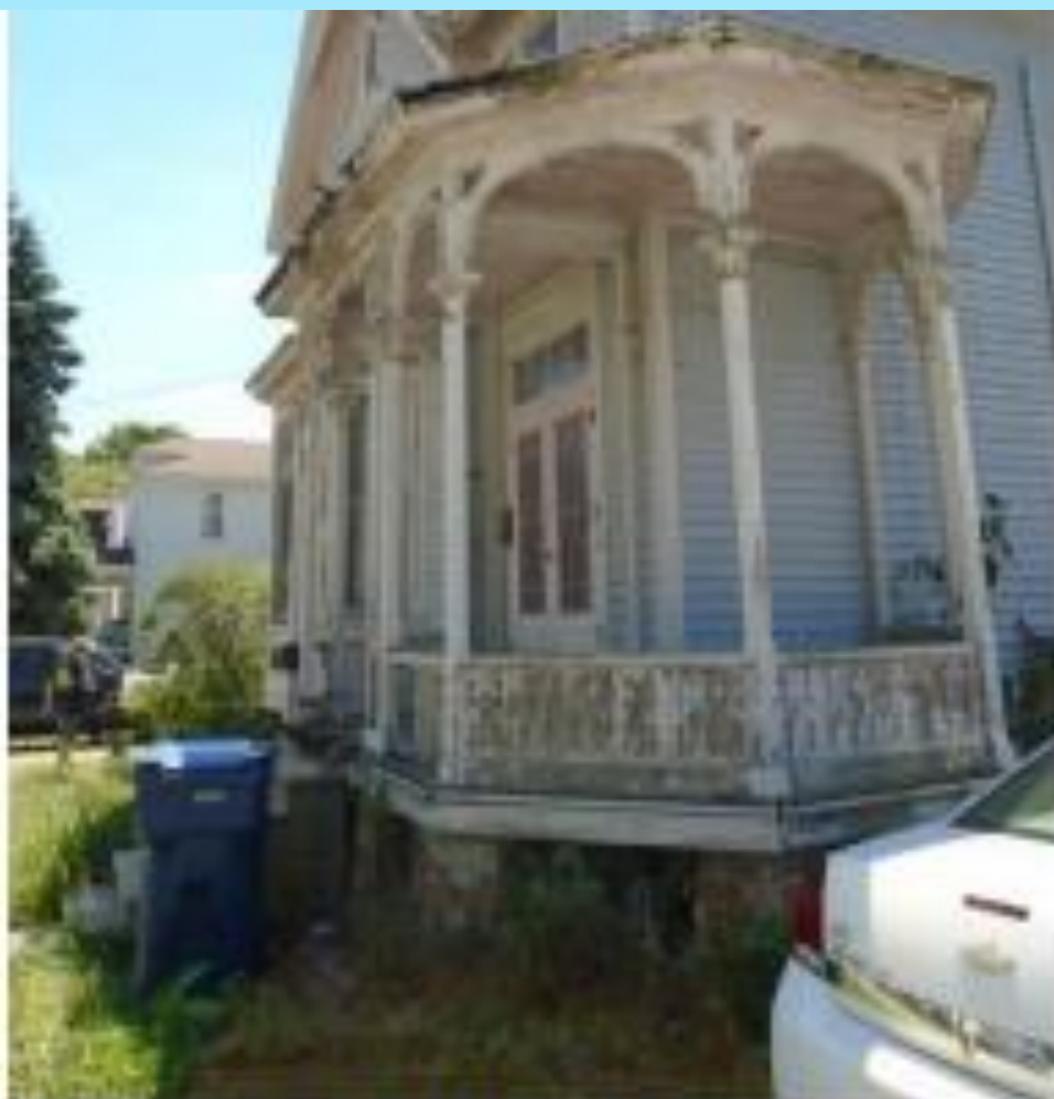
HDF-2017-5836-NEP, 521 N. Grant St., Porch Repairs BEFORE
