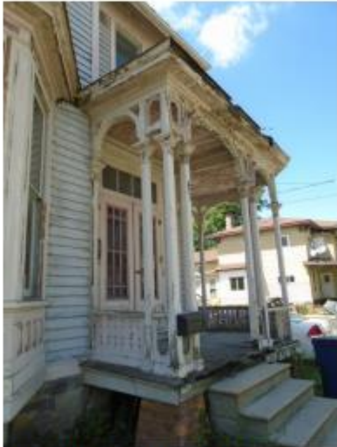
HDF-2017-5836-NEP, 521 N. Grant St., Porch Repairs BEFORE
