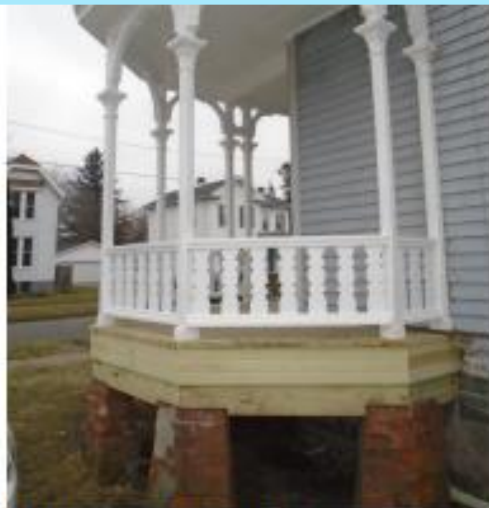
HDF-2017-5836-NEP, 521 N. Grant St., Porch Repairs AFTER
