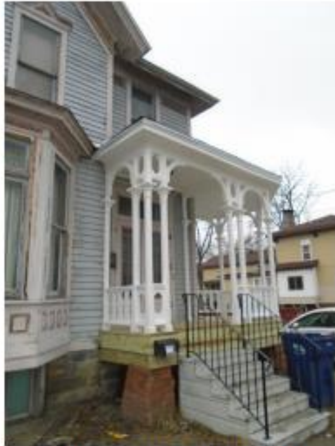
HDF-2017-5836-NEP, 521 N. Grant St., Porch Repairs AFTER
