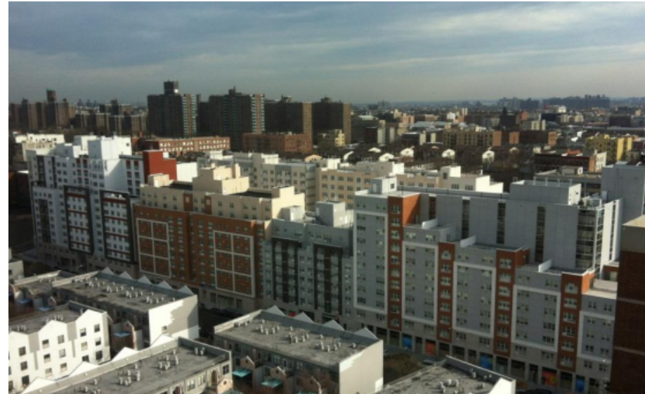
St. Ann's Terrace Fully Constructed.
