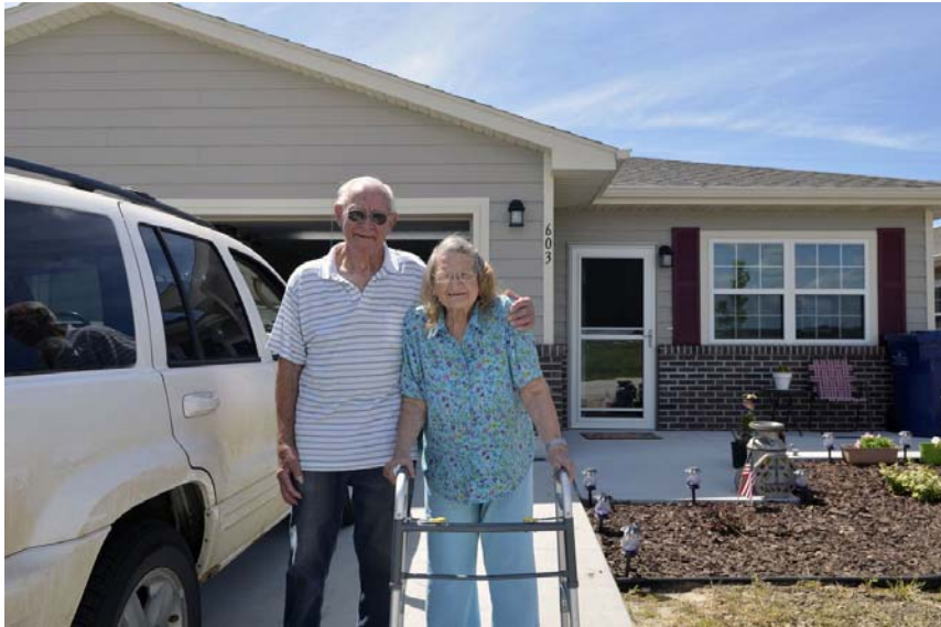
Gordon and Margaret Dunker live in one of the duplexes built through the Kracl Meadows senior housing project.
