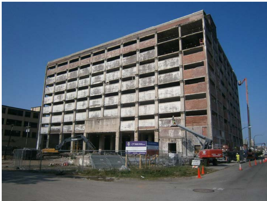
Photo circa August 2017-Demolition in progress
