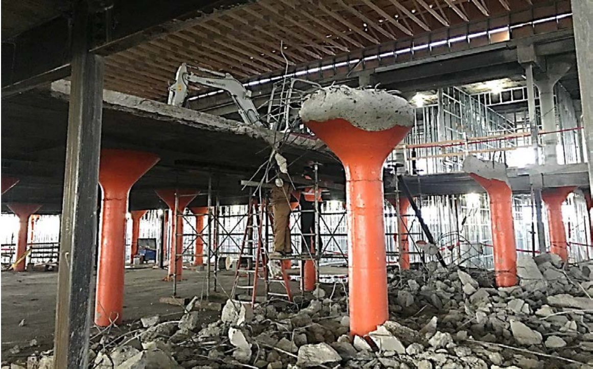
The slab is first cut to the perimeter dimension of the frame below it, and then the concrete slab is chopped away. The original concrete capital columns will be removed separately.
