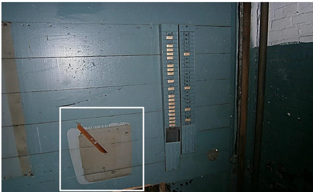
Other typical historic items for preservation: Workers Unemployment Insurance Notice (above) and a time card slot below. The highlighted box is where the time clock was.
