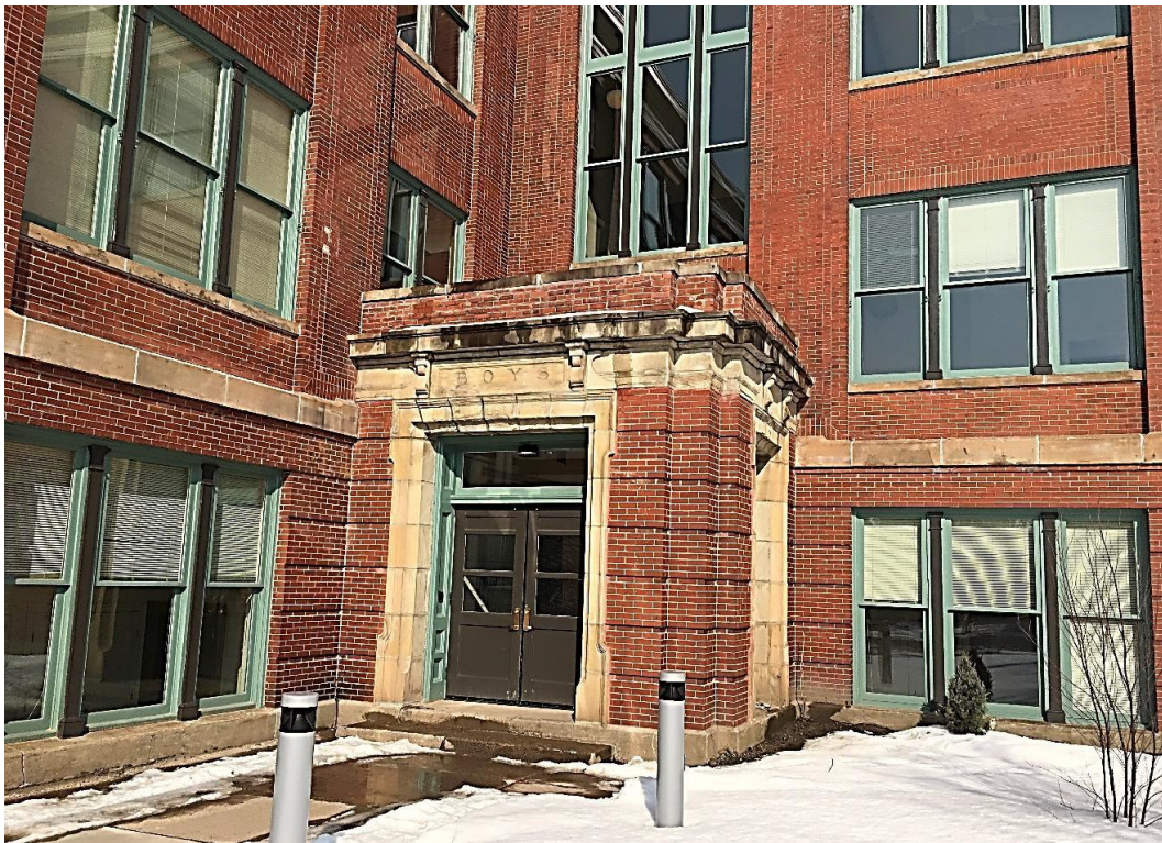
Restored Girls and Boys entrances. These are now mainly used for emergency egress
