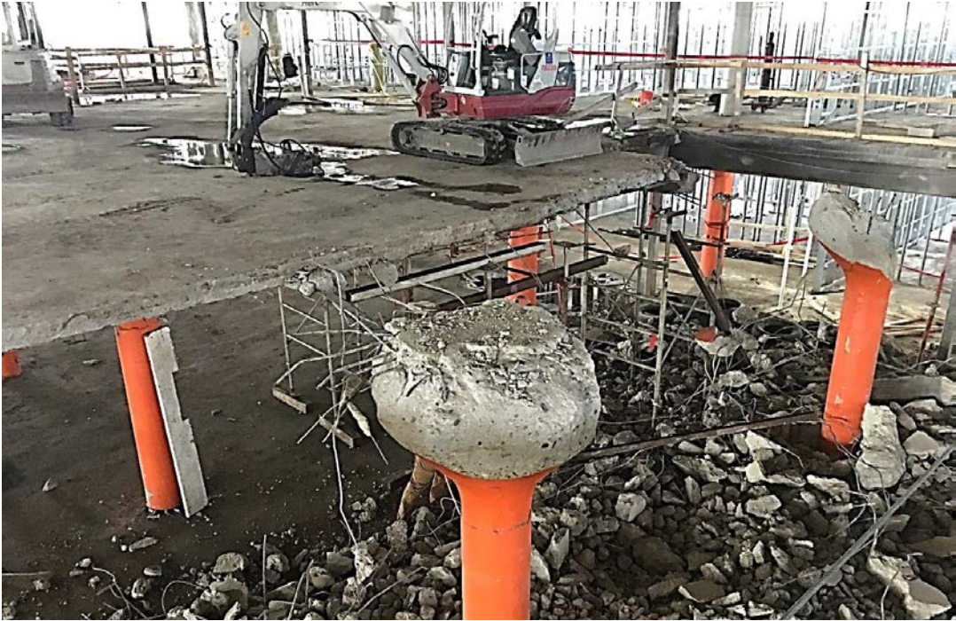
The slab is first cut to the perimeter dimension of the frame below it, and then the concrete slab is chopped away. The original concrete capital columns will be removed separately.
