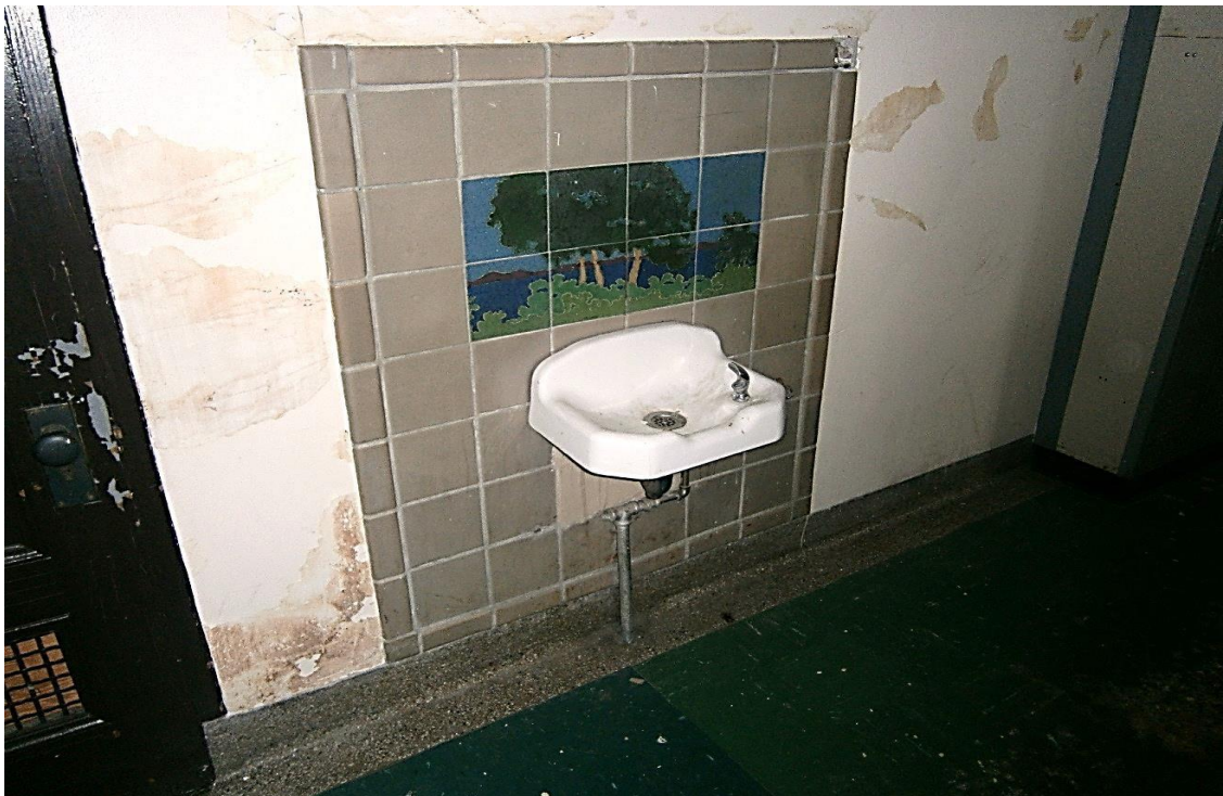
Typical historic elements to be preserved include the decorative tile reliefs over drinking fountains which are believed to have been done as a project by students after the school opened.
