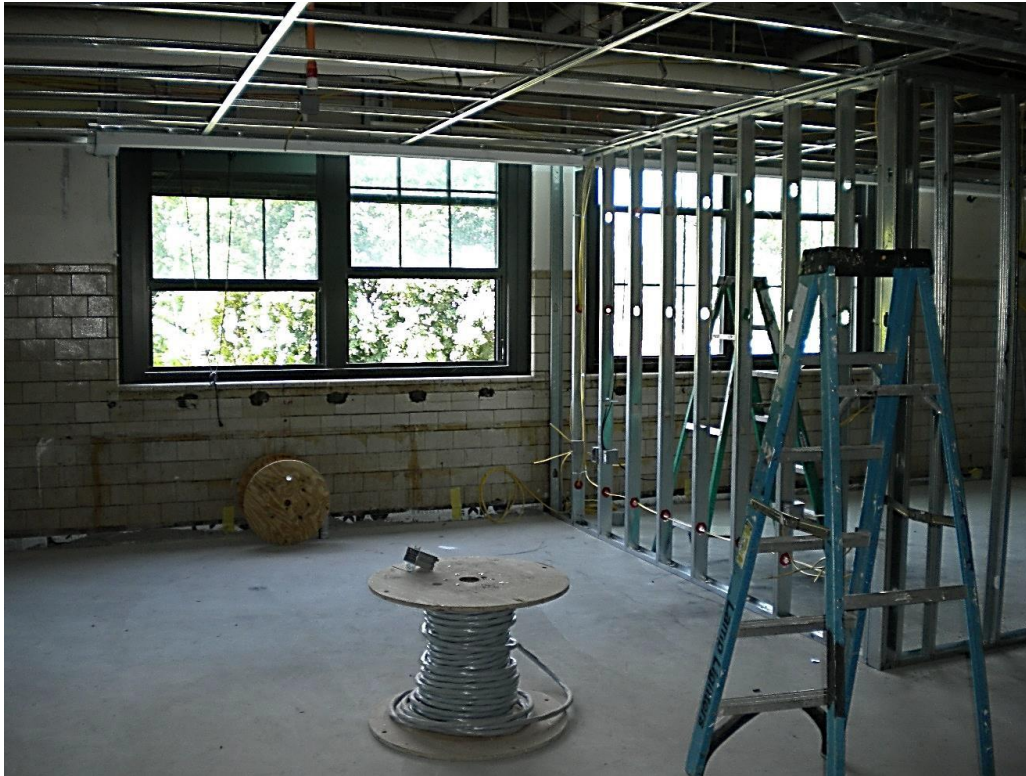
Upper level apartments in progress with new replicated windows
