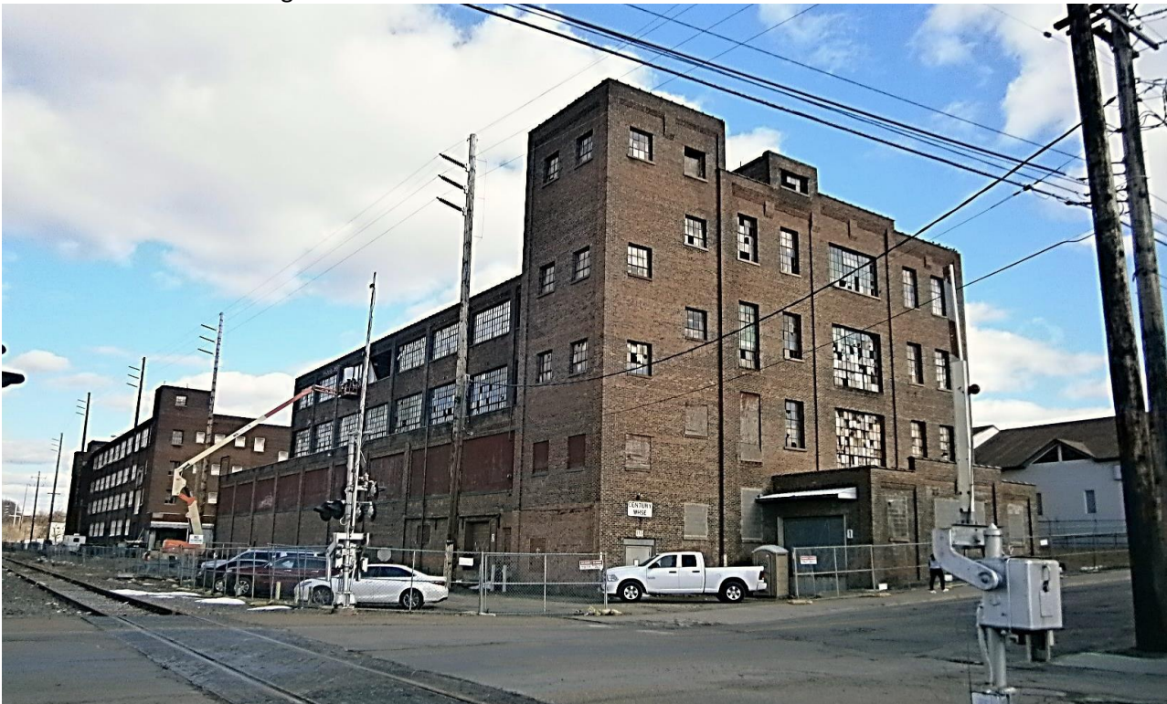
Work commenced March 20, 2017
