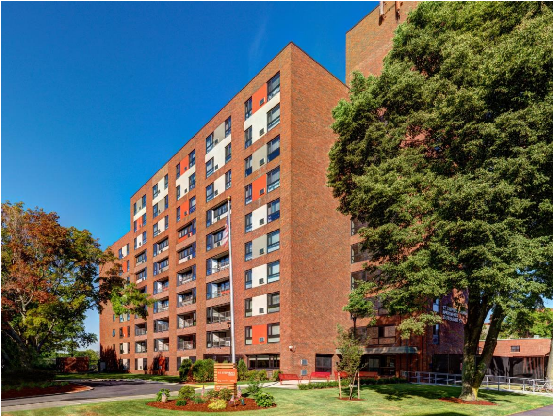
Photo: St. Stephen's Tower
