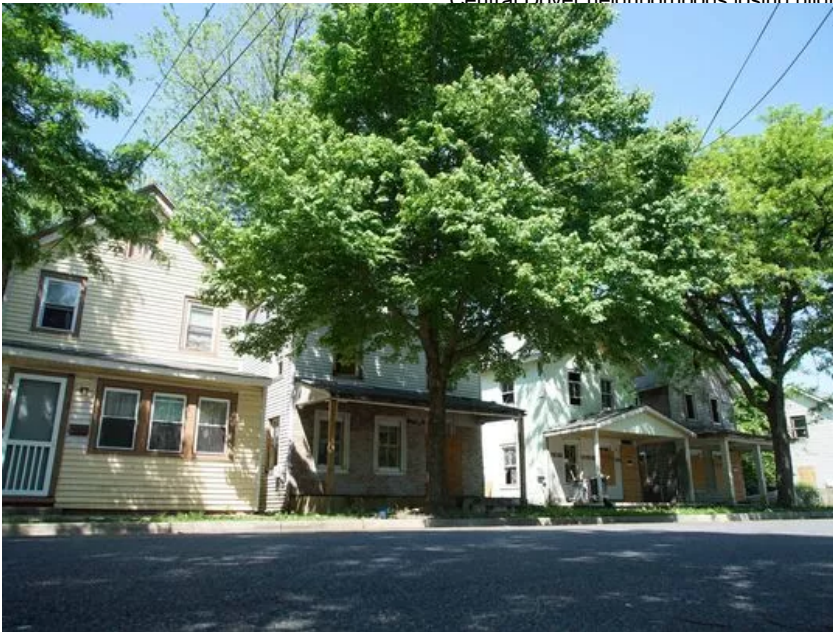
Five properties along North Kirkwood Street in Central Dover will be torn down and four new homes built in an effort to increase homeownership in Central Dover neighborhoods. (Photo: Jennifer Corbett, The News Journal)
