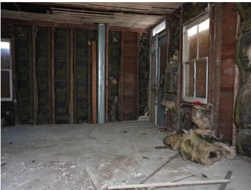
An interior of a property along N. Kirkwood St. The property will be demolished and rebuilt by Strong Neighborhood Housing Funds near downtown Dover in an effort to stop blight and improve housing. (Photo: Jennifer Corbett, The News Journal)
