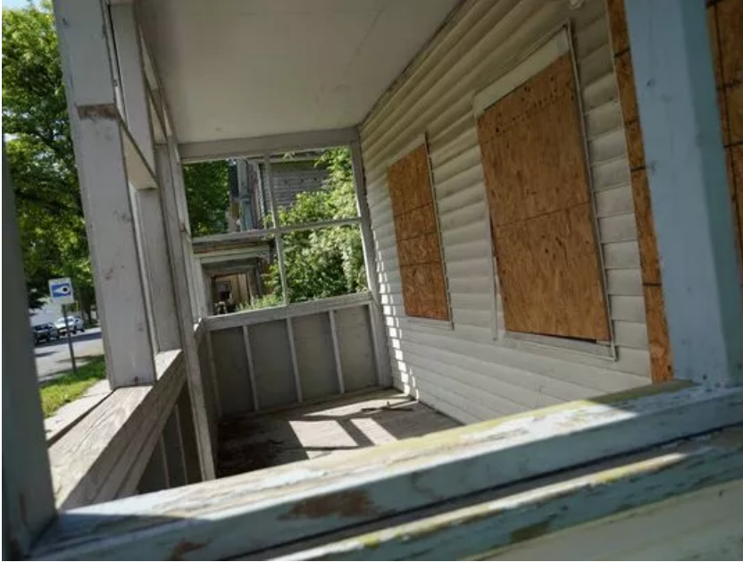
Properties along N. Kirkwood St. wait for demolition and will be rebuilt by Strong Neighborhood Housing Funds near downtown Dover in an effort to stop blight and improve housing. (Photo: Jennifer Corbett, The News Journal)
