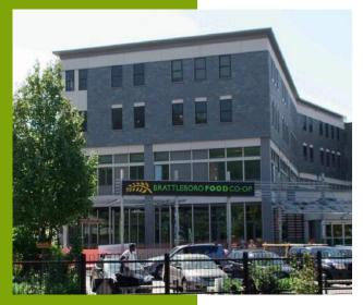
Construction materials included locally harvested and milled flooring and slate siding manufactured in Vermont. Green features have cut costs by approximately 50 percent, which helps keep the apartments affordable and saves 21 tons of CO2 emissions a year.
