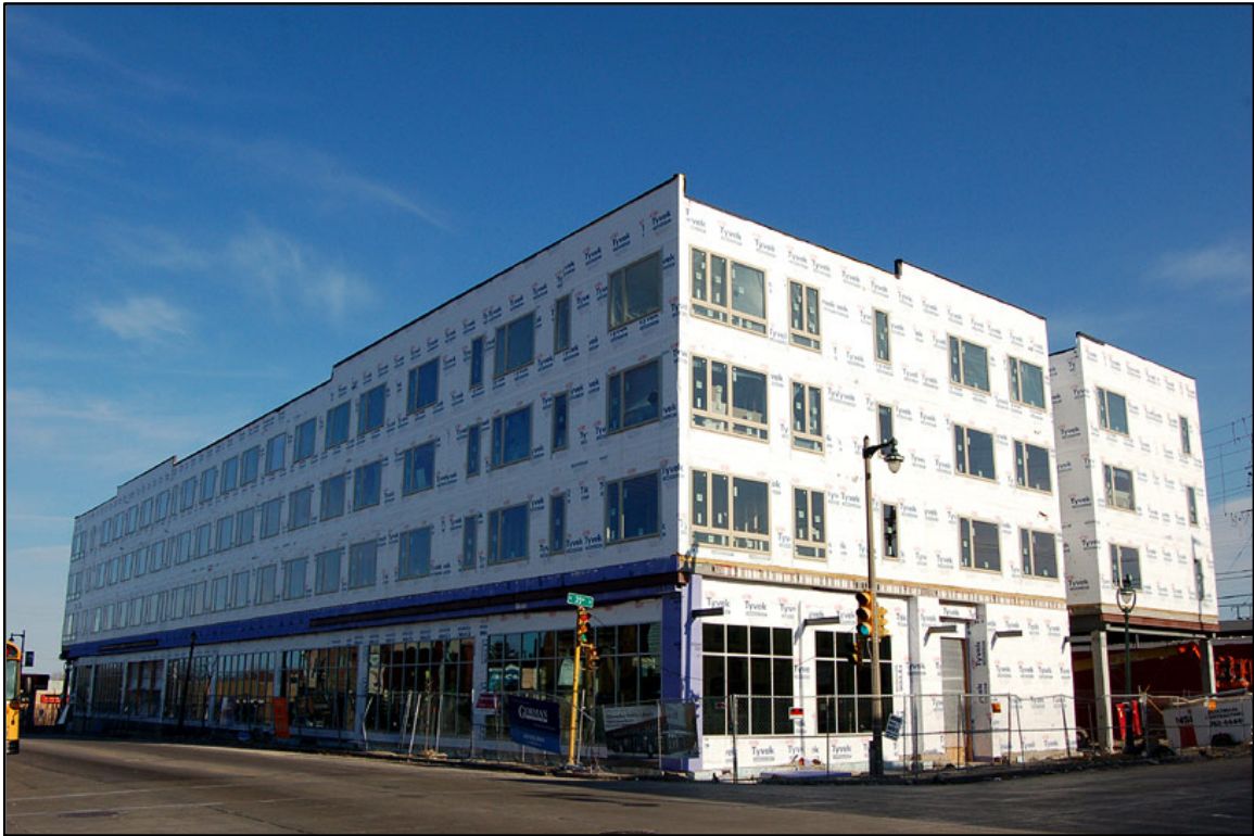
Villard Square Construction
