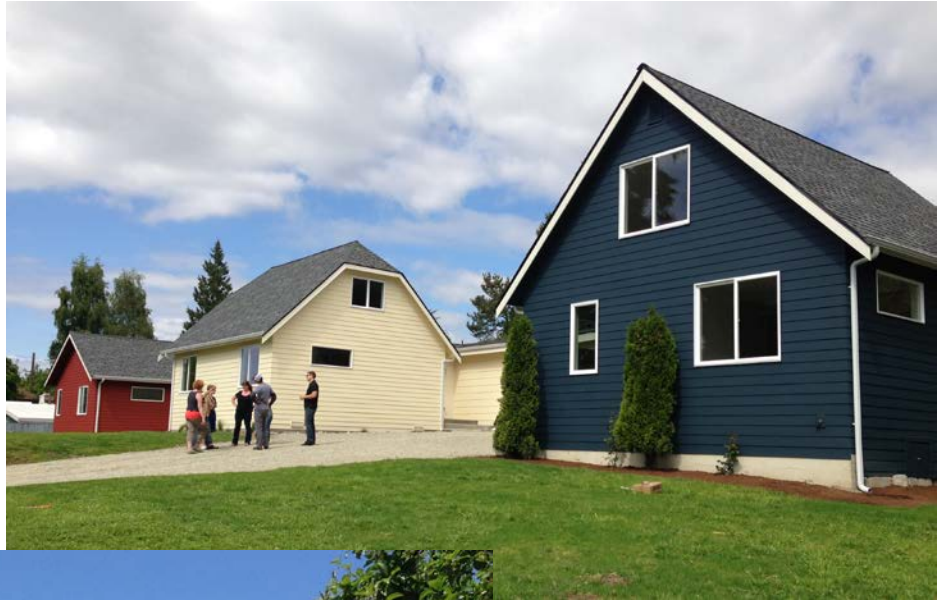
The Triplets—three homes rebuilt by Green Canopy Homes with support from the Housing Finance Commission.
