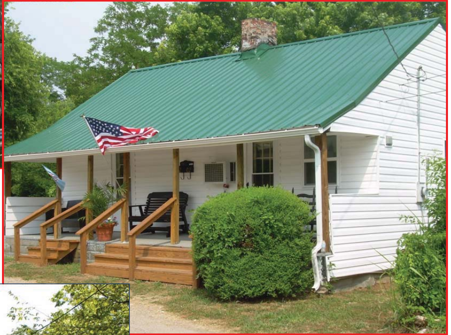
Johnny Scribner's Columbia home, before and after Emergency Repair Program assistance through People Helping People Together.
