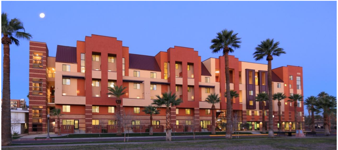
Urban Living on 2 nd Avenue - Phoenix, Arizona
