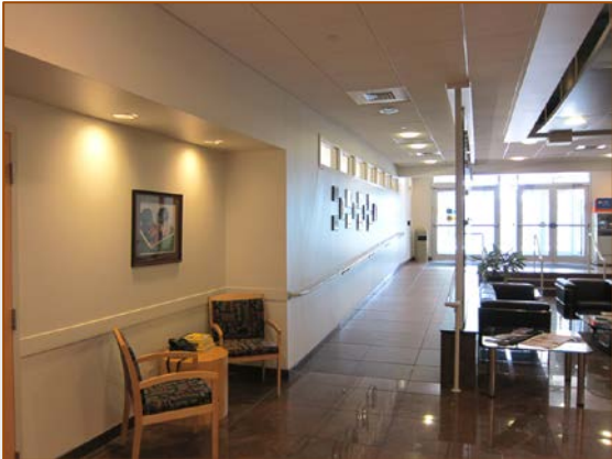
PHFA lobby prior to story wall installation
