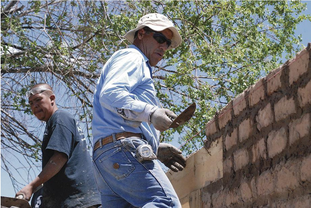
Workers use new mud and old adobes
