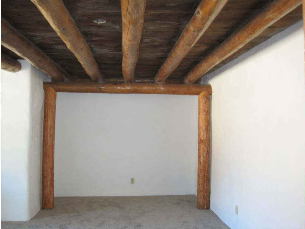
Preserving the vigas (exposed roof beams) and ceiling is a high priority
