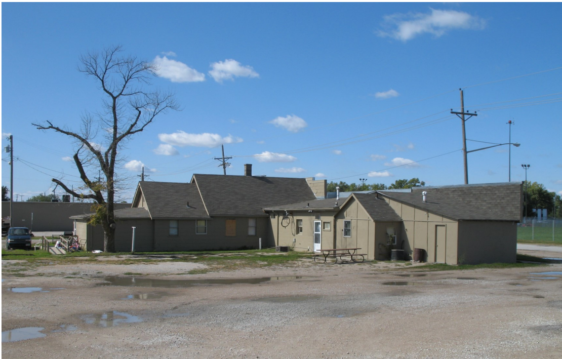
Rebuilding Lives Center - BEFORE
