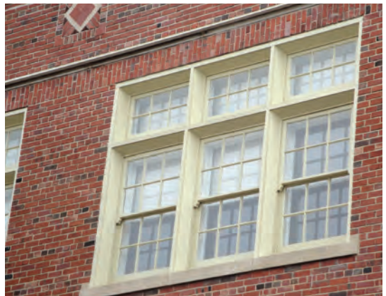
A before and after look of windows at the DCHFA-financed House of Lebanon senior apartments.
