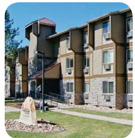
Aspenwood after renovations.
