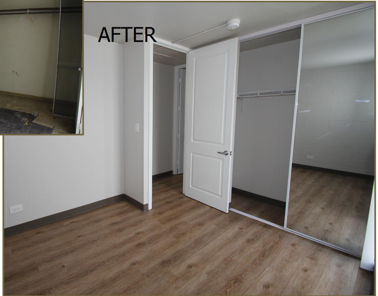
BEDROOM RENOVATIONS: wire shelving in closets and mirrored bypass closet doors
