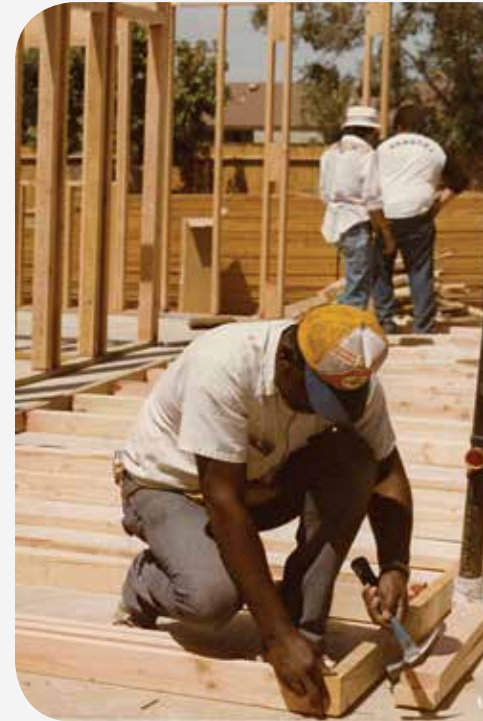
SELF-HELP BUILDER CONSTRUCTING A NEW HOME
