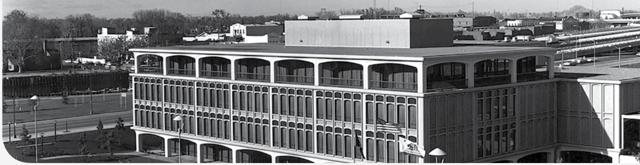
CALHFA'S FIRST OFFICE AT 300 CAPITOL MALL, SACRAMENTO
