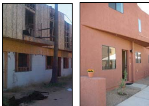
▶ Before and after photos of units at Glenn Verde.
