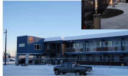
Karluk Manor Anchorage, Alaska
