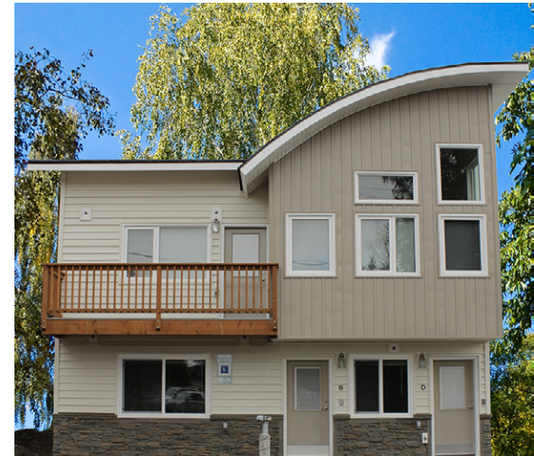
1248 East Ninth Avenue four-plex project in Anchorage.
