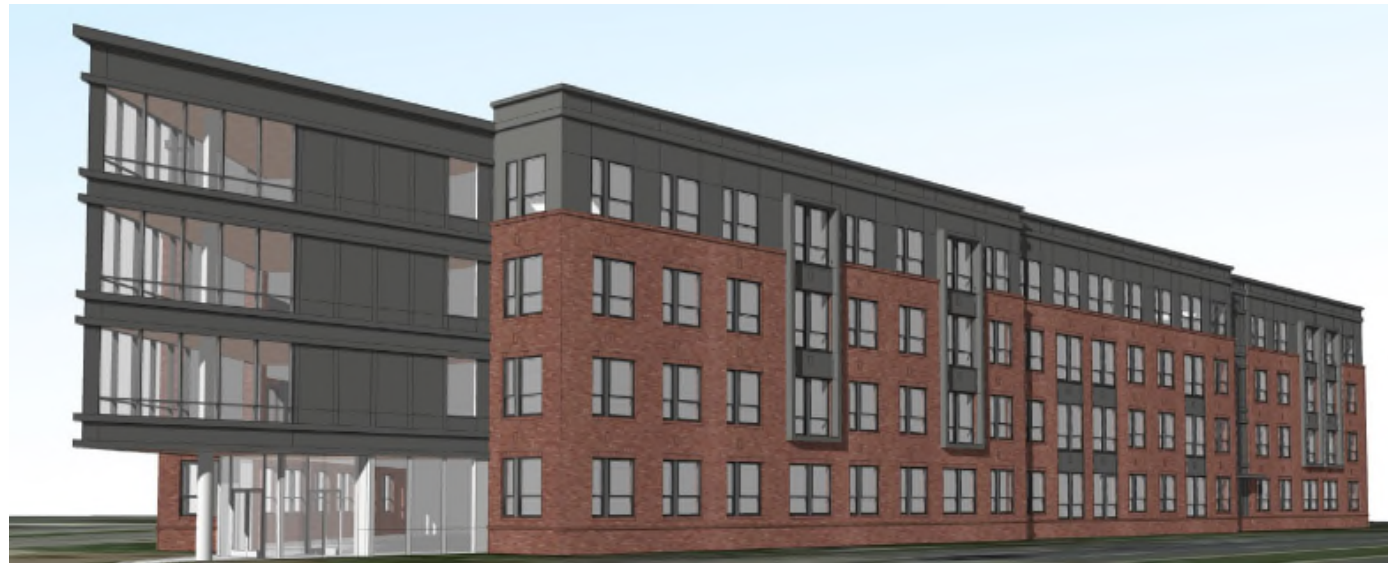
Metro Heights (Maryland)
